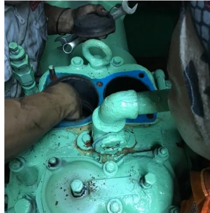
Gambar 4. Pemecah low pressure suction valve
